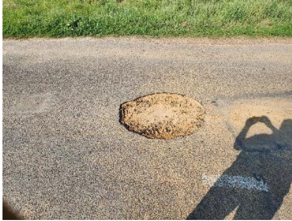
Pic 5: Saxonwold Road Distress - Potholes
