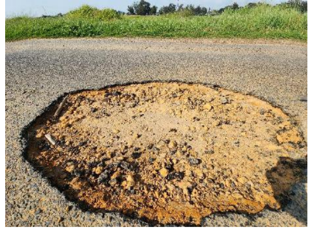
Pic 6: Saxonwold Road Layerworks Laterite
